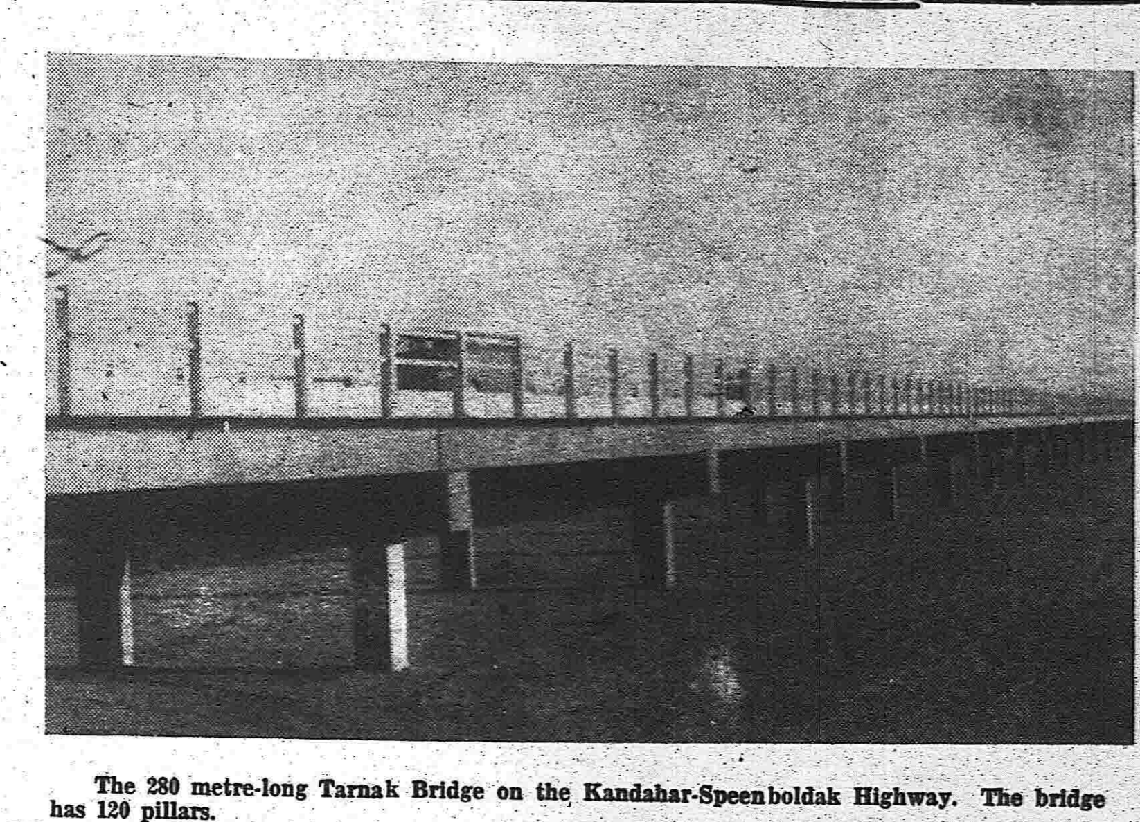
The 280 metre-long Tarnak Bridge on the Kandahar-Speenboldak Highway. The bridge has 120 pillars.
