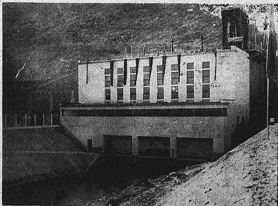
Utilization of electric power is one of the main goals of our revolutionary government. Photo shows a power station in the country.
