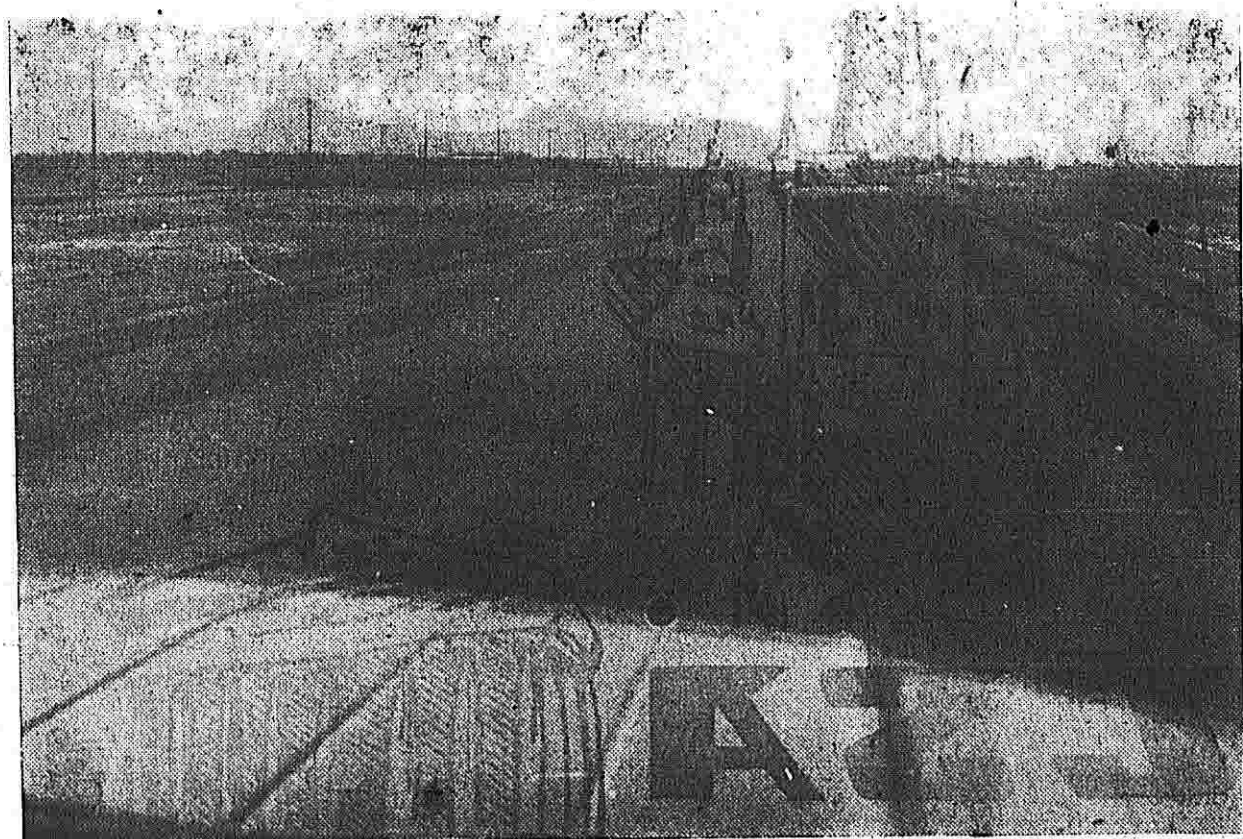
Here is the completed road. The total width of the road is 10 metres while that of the pavement is seven metres.
