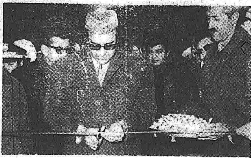
Eng. Reza dedicating the Khoram canal headworks.
