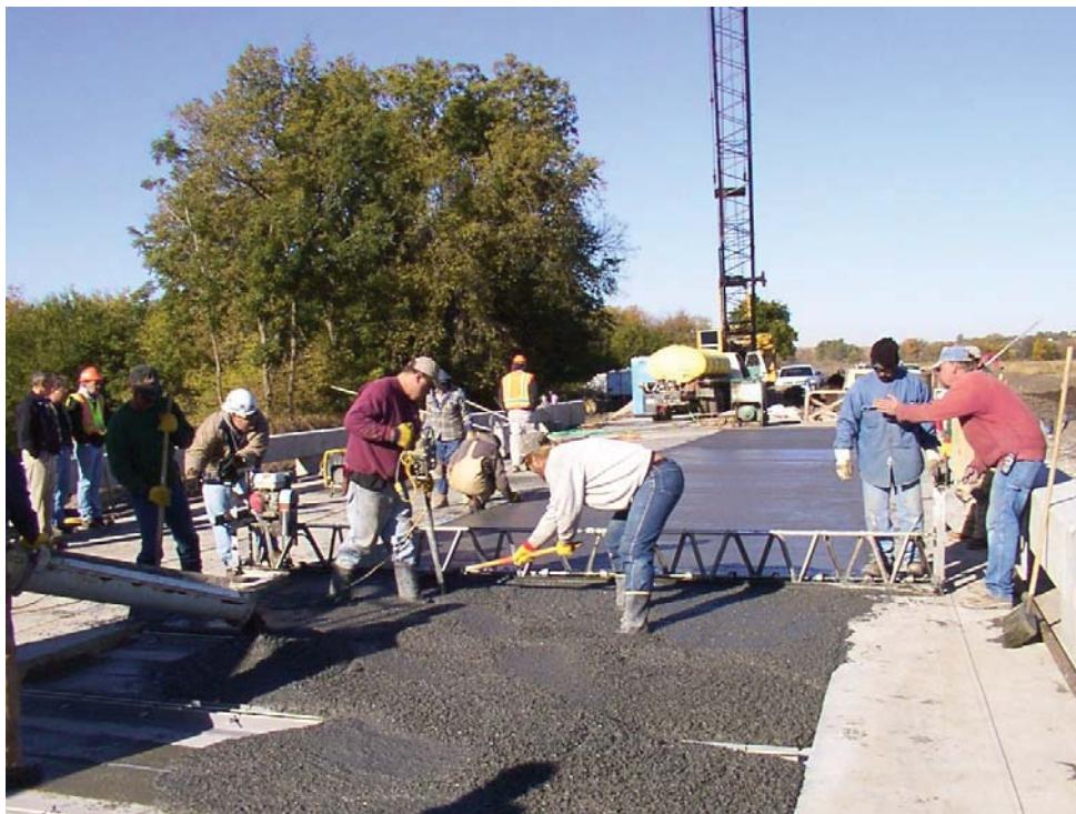
FIGURE 9 Casting the westbound lane with conductive concrete.
