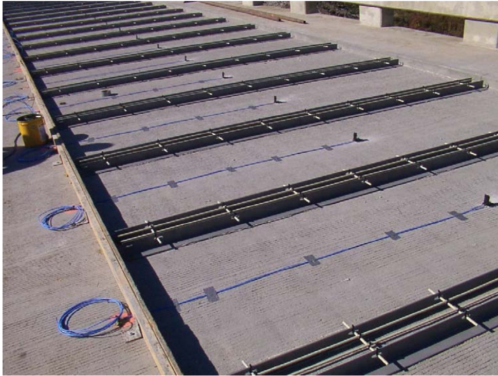
FIGURE 8 Electrode layout during construction.
