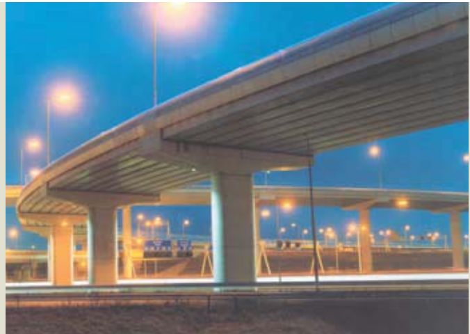
Figure 1. A curved, pretensioned concrete box-girder bridge in Rotterdam, Netherlands, is a prime example of standard practice for bridges in the Netherlands for more than a decade. Courtesy of Spanbeton.
