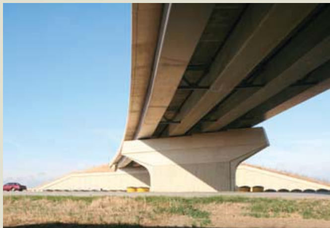
Figure 6. The Arbor Road Bridge in Lincoln, Neb., is a two-span, horizontally curved, precast concrete-girder bridge with a skew of 31 degrees and a central angle of about 3 degrees.
