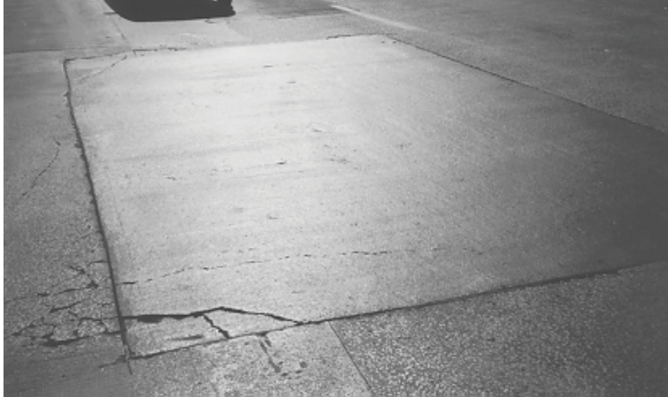
Figure 1. Conductive concrete patch after 12 months
