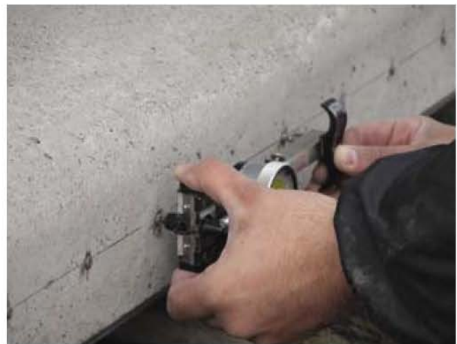
Fig. 9. Transfer length measurement.
