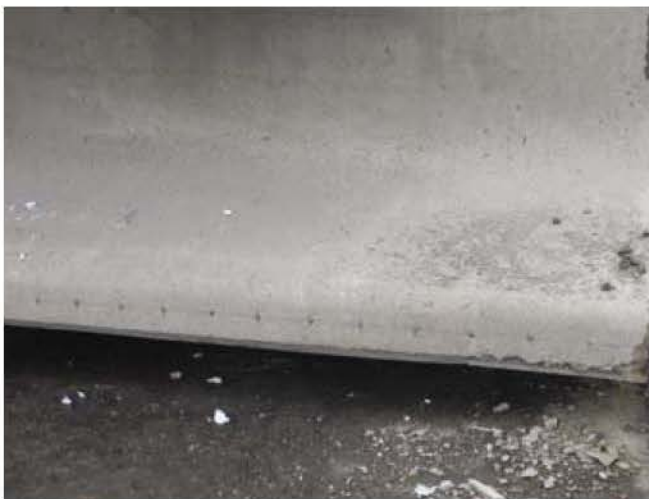
Fig. 8. Demec point locations and beam end.
