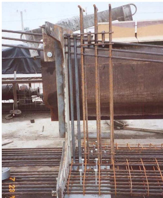
Fig. 14b. Proposed end zone detail NU1100 I-girder NU1100 I-girder.
