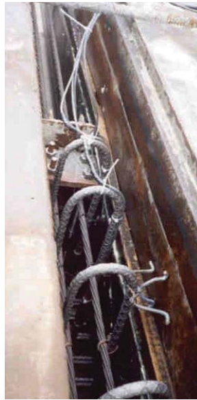
Fig. 10b. Shear reinforcement placed after the end zone reinforcement – IT400.
