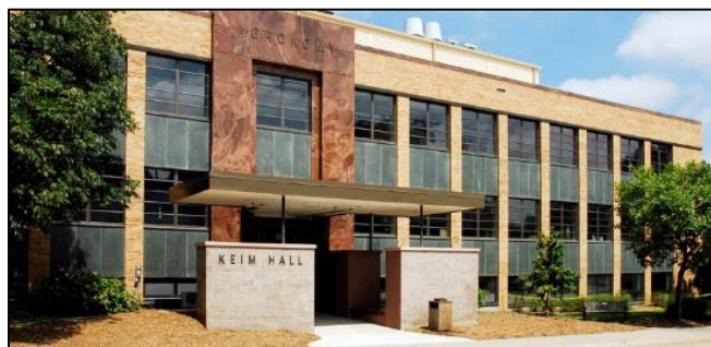
Keim Hall at UNL, where renovation of classes, labs and offices resulted in improved learning and teaching space.
