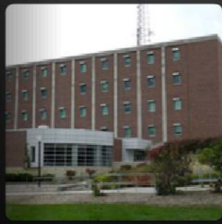
Allwine Hall (AH) SCIENCE FACILITY
