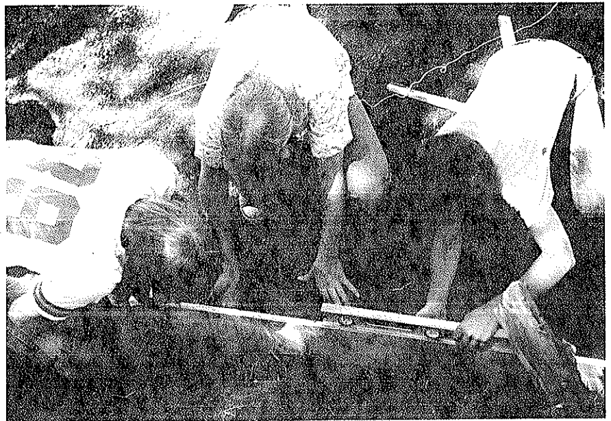
FIGURE 3. Students aided teachers and various community, state, and federal resource groups in completing many pond projects. This young trio is constructing a concrete slab for an outdoor cooker.
