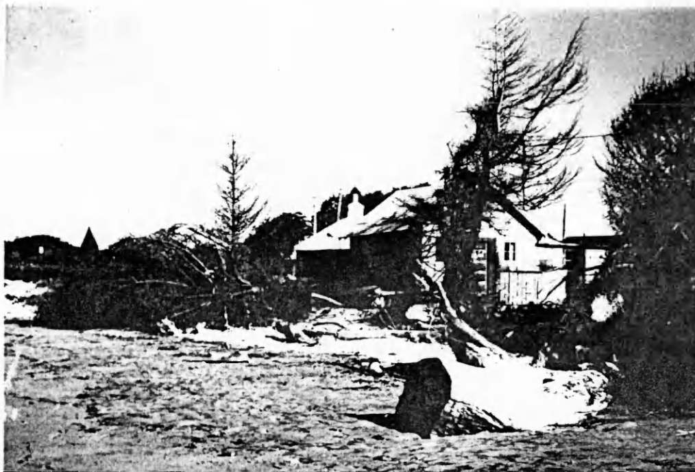
Photograph 8. These bayfront cottages on Maple Street and other homes nearby have been damaged by floodwaters in recent years due to erosion of the bay beach prompted by construction of a groin immediately upstream from the area.
