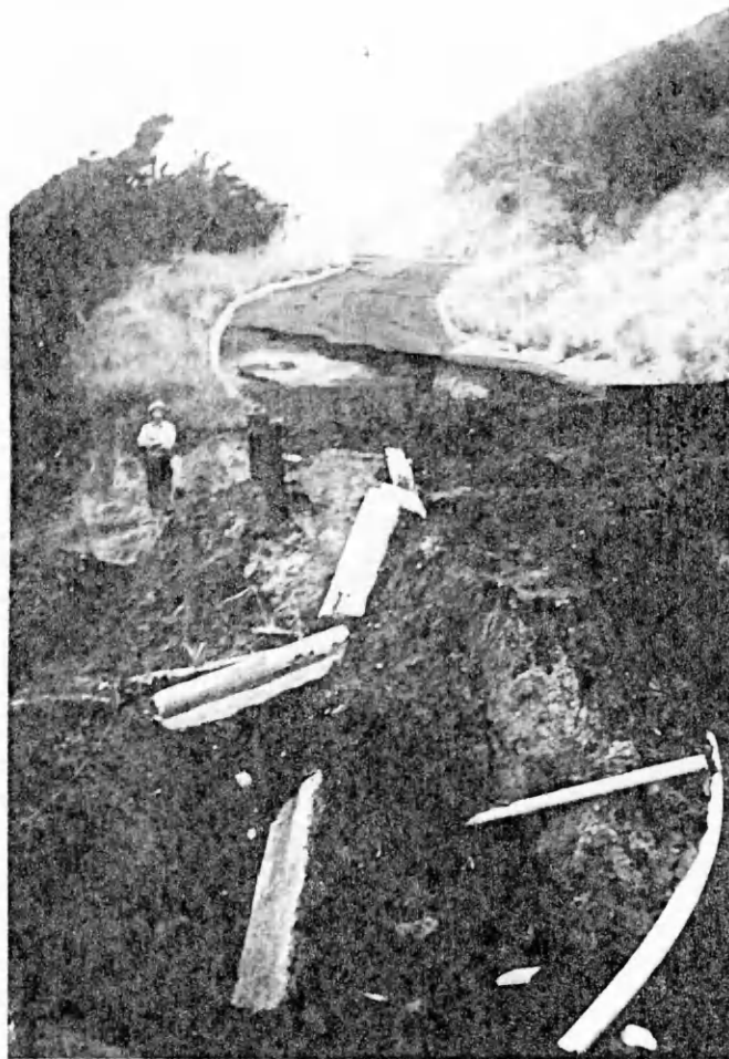
Photograph 5. Road cuts or other construction-related disturbance can oversteepen a slope or burden slide-prone materials to the point of failure. This site is a particularly sensitive hazard area in north Newport. Newly constructed roads, a retaining wall, sewer and water lines and underground cables were extensively damaged in this expensive lesson in coastal geomorphology.
