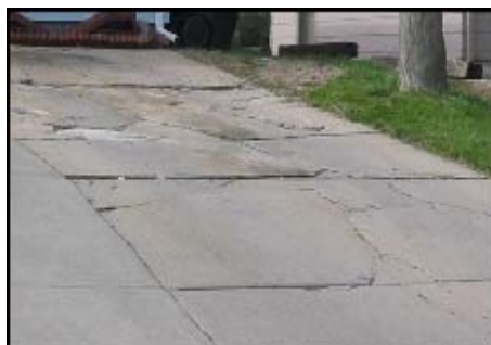
Major problem. Cracks with edges that are even or higher on one side
