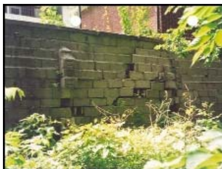
Minor problem. Wall is missing pieces, crumbling.
