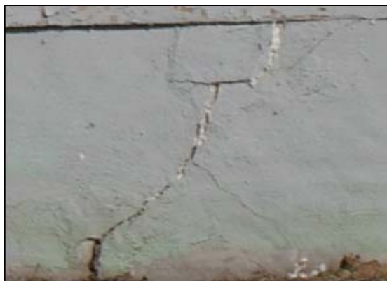
Minor problem. Hairline crack, loose and flaking mortar. Covering less than 25% of the foundation walls.
