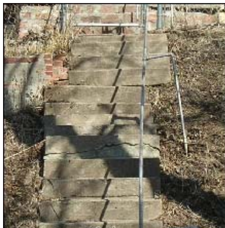
Major Problem. Major problem. Loose or missing concrete/ boards, cracks and holes,
