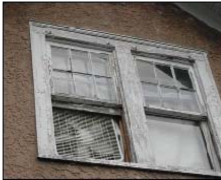
Minor problem. Less than 25% of window pane is cracked or broken.
