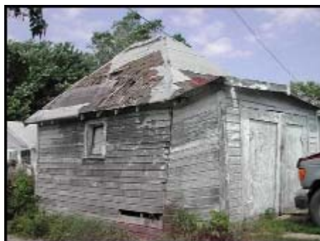
Major problem. Roof problems, rotting siding/boards, structure needs painting, structure looks slanted/not level
