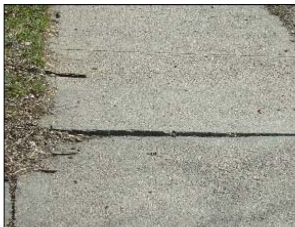
Minor problem. Cracks with edges that are evident; cracks do not present a walking or other hazard.
