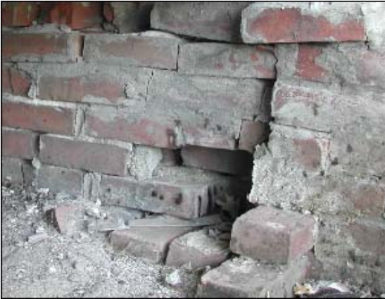
Major problem. Settling, bulges in foundation wall, crumbling material & holes.
