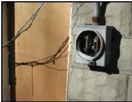
Major problem. Exposed wires, broken bulbs and fixtures, exposed socket.
