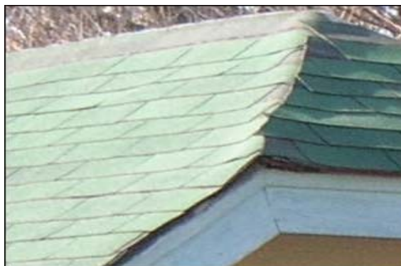
Minor Problem. Sagging roof ridge line, structural deterioration.
