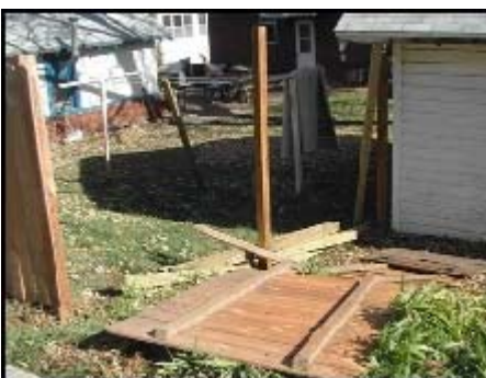
Major problem. Fence is broken, slanted and missing pieces.
