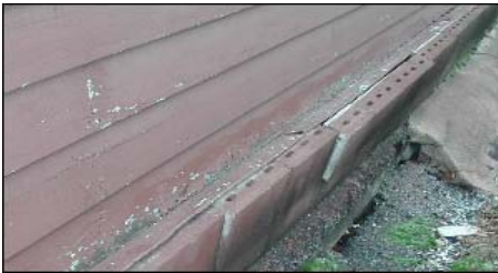
Major problem. Missing parts & lacks a section of foundation.
