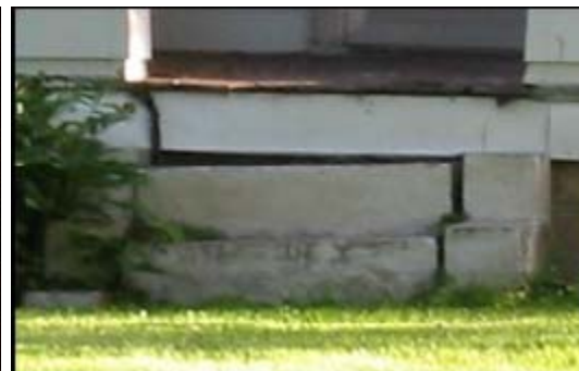
Major Problem. Major problem. Loose or missing concrete/ boards, cracks and holes,
