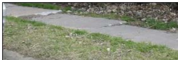
Minor problem. Cracks with edges that are evident; cracks do not present a walking or other hazard.
