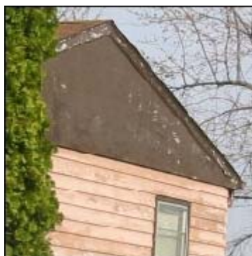
Minor Problem. Cracking, blistering, peeling of paint and/or bare wood less than 25% of the exterior surface.
