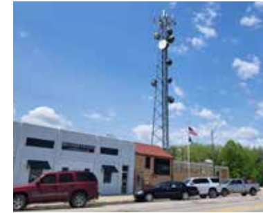
Ainsworth Cell Tower
