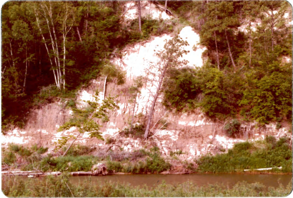
A. Failure of slope.
